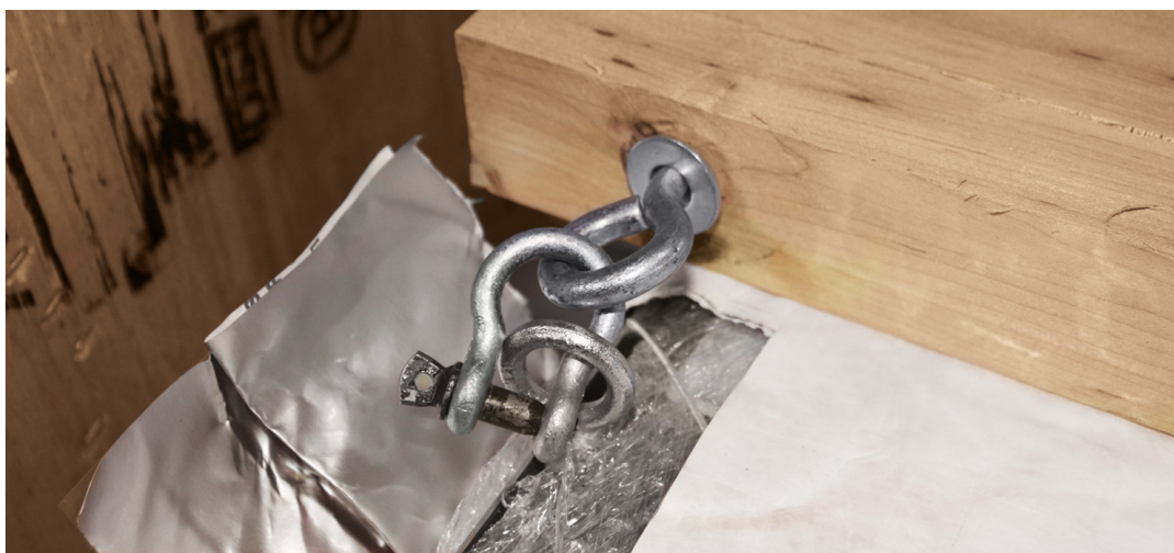
Figure 4-14. Attaching Eye-bolts to Spreader Bar
